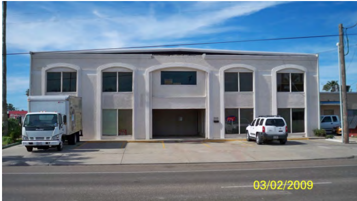
View off of highway 100
